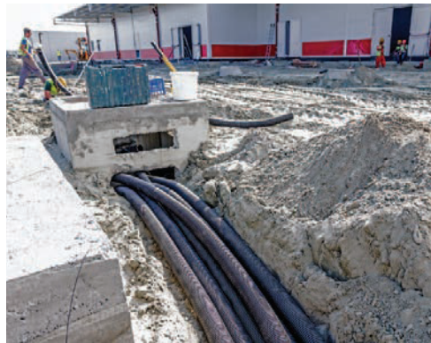
Example of bulk installation of conduits
