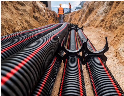
Example of installation using spacers between conduits
