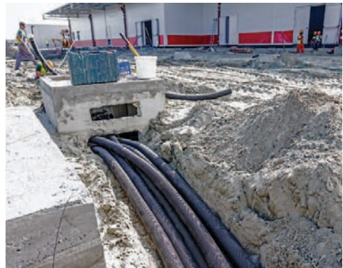
Example of bulk installation of conduits
