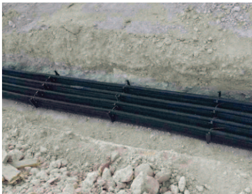
Example of installation using spacers between conduits
