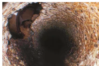
Cement pipes are very vulnerable to chemical attacks and specifically to sulphuric acid, therefore a lot of wear is observed as time passes !
